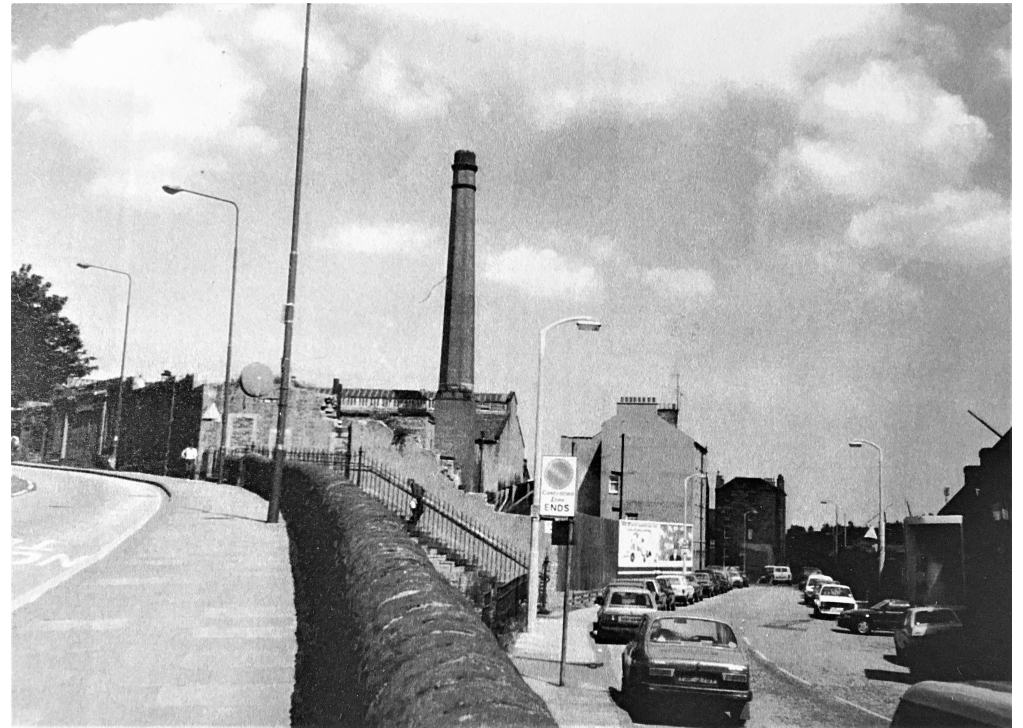
VIEW OF ABBEYHILL CLOSE TO GRAHAM CHATHAM'S BUSINESS
