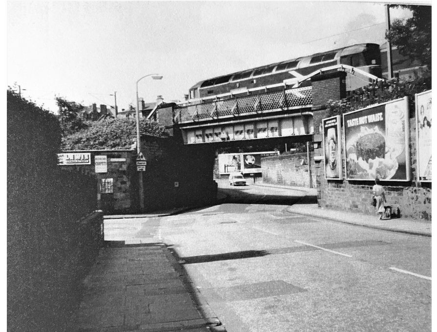
VIEW OF ABBEYHILL CLOSE TO GRAHAM CHATHAM'S BUSINESS
